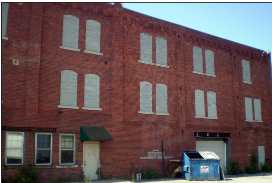
This 18th century era factory on West Auburn Avenue in Bellefontaine was once used to manufacture hearses. Tri-County Community Action has received a grant from the Ohio Department of Transportation to demolish most of the building and refurbish its salvagable portions as a facility for its Logan County transportation program. The $2.6 million grant will help revitalize the neighborhood.
