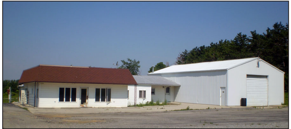
This complex of four buildings on County Road 130 near Bellefontaine is no longer empty thanks to Tri-County Community Action. The agency moved its Home Weatherization Assistance Program into the complex June 29.
