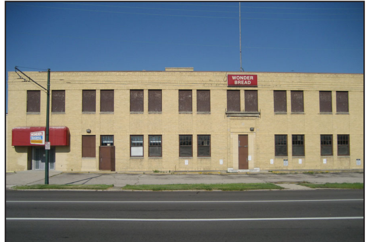
CAP Dayton's HWAP program is gradually moving into this former bakery at 947 Ludlow Street in downtown Dayton. The bakery has been empty for several years. An outlet store closed shortly before the agency purchased the building in 2008.
