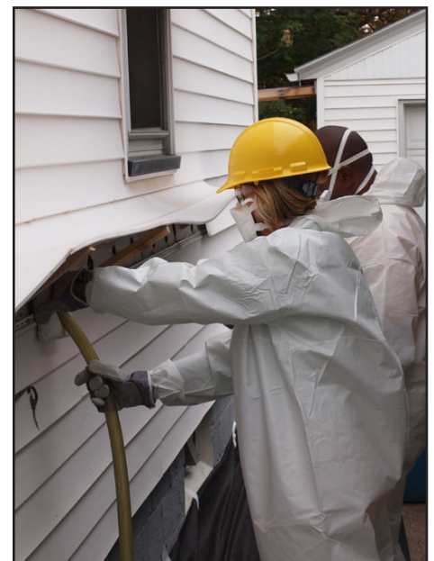
Congresswoman Betty Sutton works with Milton Card from the Lorain County Community Action Agency to blow cellulose insulation into the sidewall of Rosa Kimbrough’s 1950s home in Lorain.
